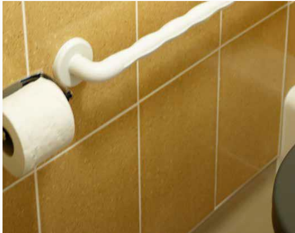
A good example of contrast so that person can see handrail
